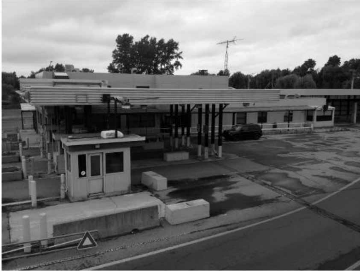
fig. 25 - Cornwall Island Customs Building, before demolition, image from Public Works and Government Services of Canada Project Report: "Demolition of former Customs Buildings, Cornwall Island, Ontario", May 2015
