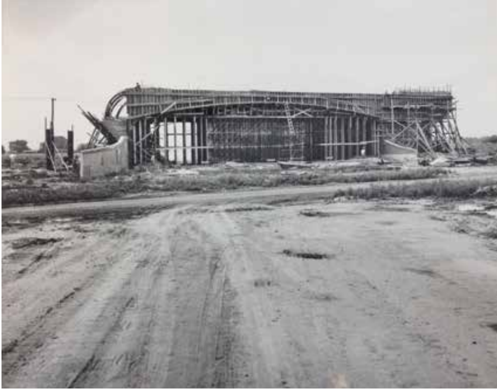
fig. 8 - Underpass Construction, Highway 401, Chatham, July 26, Archives of Ontario
