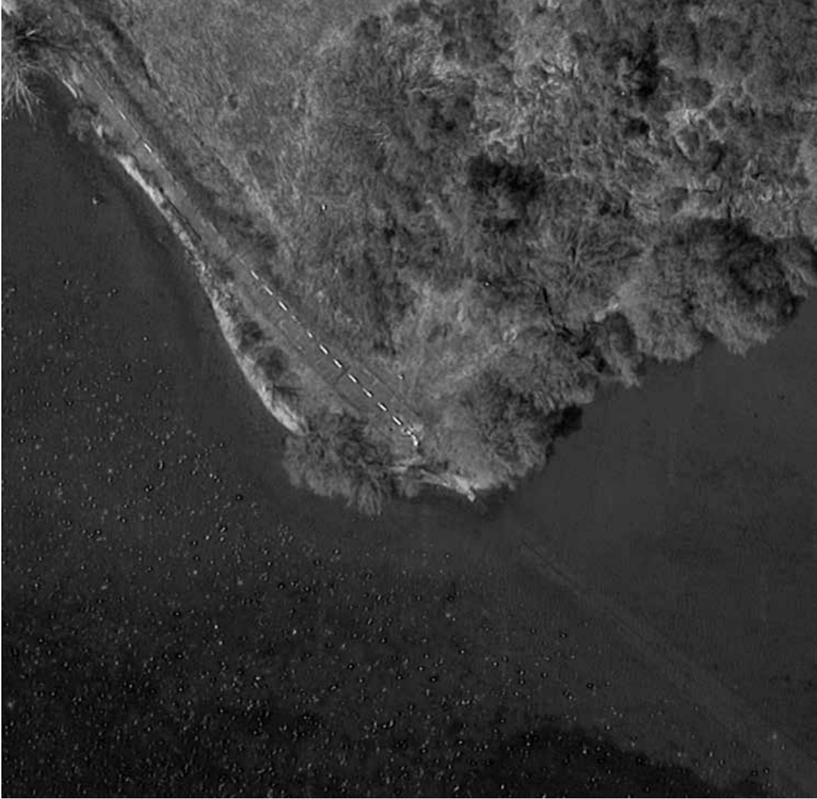
fig. 26 - Broder Island, with view of submerged King's Highway No. 2, South Dundas, Ontario, Google Earth View, 2015
