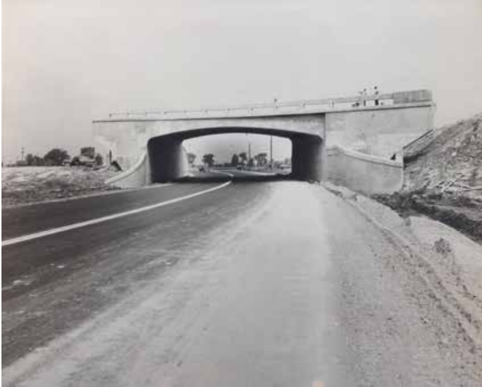
fig. 9 - Overpass Construction, Highway 401, Chatham, July 26, 1956, Archives of Ontario
